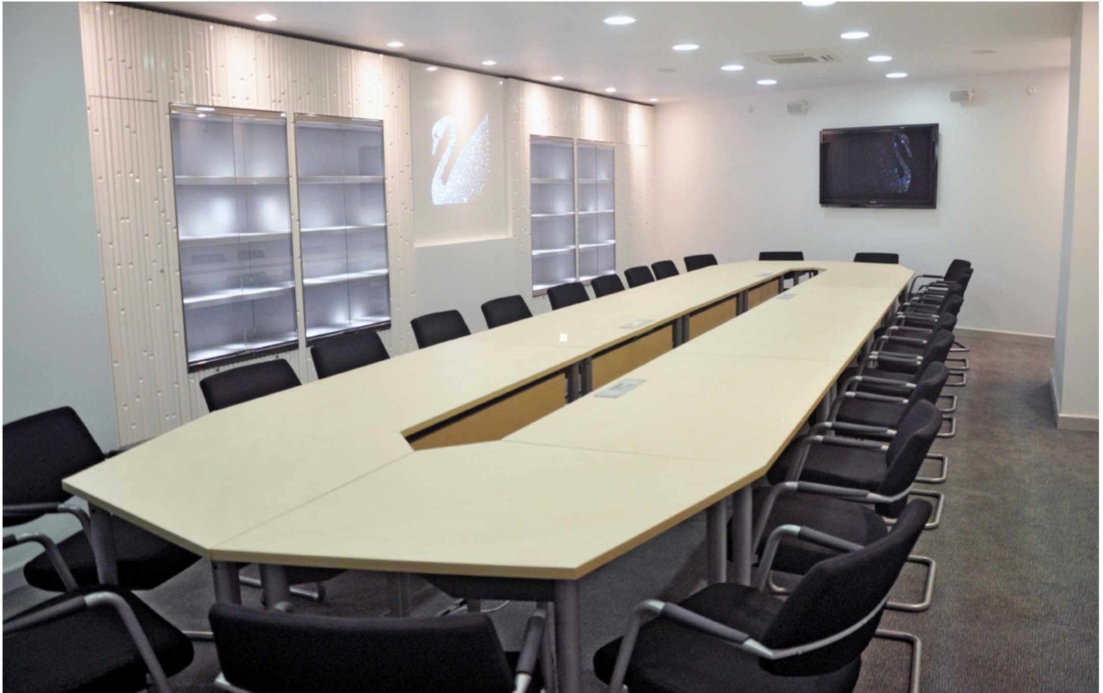
Pop-up power and data unit installed at Swarovski, London, UK.
